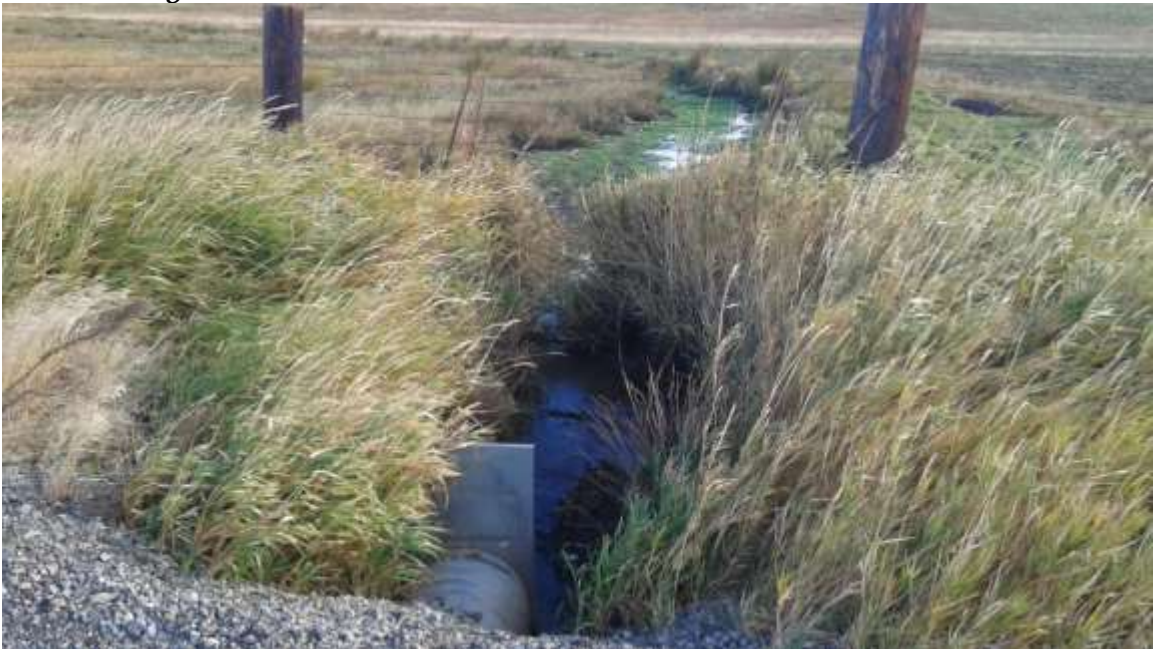
Above and below: The main irrigation ditch that drains onto on the northeastern corner of the site, east of Lower Green Canyon Road. Note control structure to shut off flow of irrigation water to the west of Lower Green Canyon Road.
