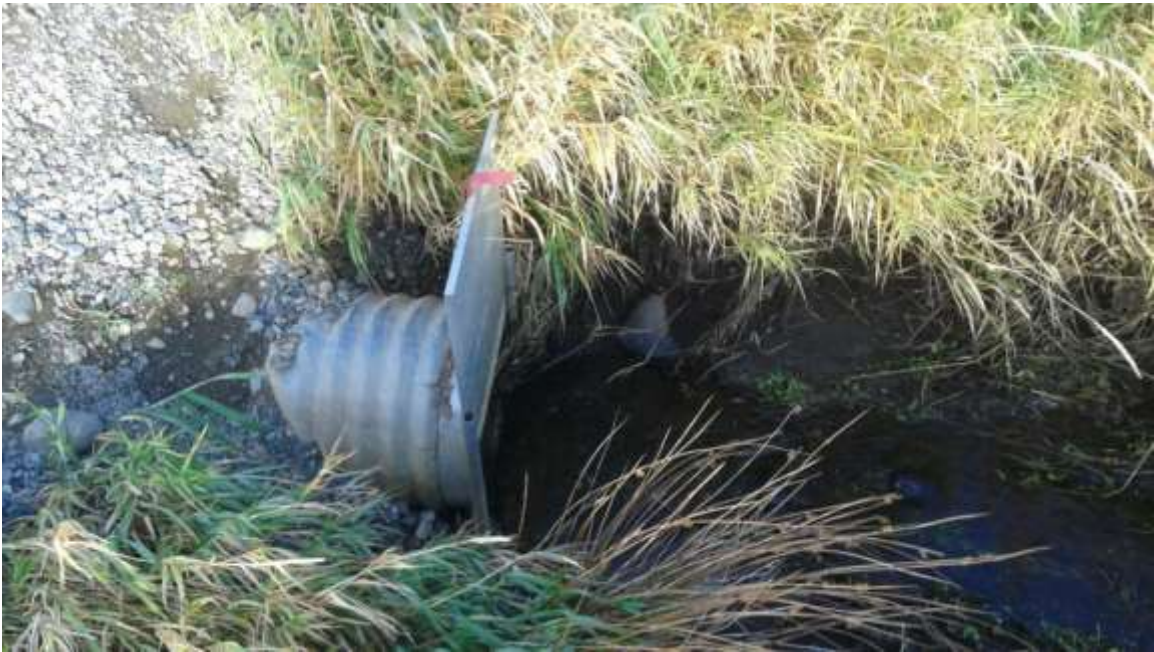
Above and below: The main irrigation ditch that drains onto on the northeastern corner of the site, east of Lower Green Canyon Road. Note control structure to shut off flow of irrigation water to the west of Lower Green Canyon Road.
